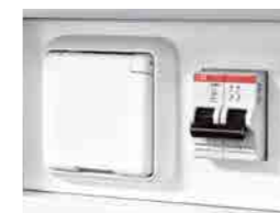
Electrical break automat
